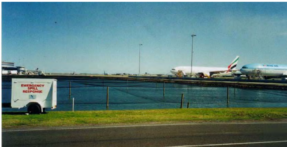
Bird netting over ponds at Sydney Airport
