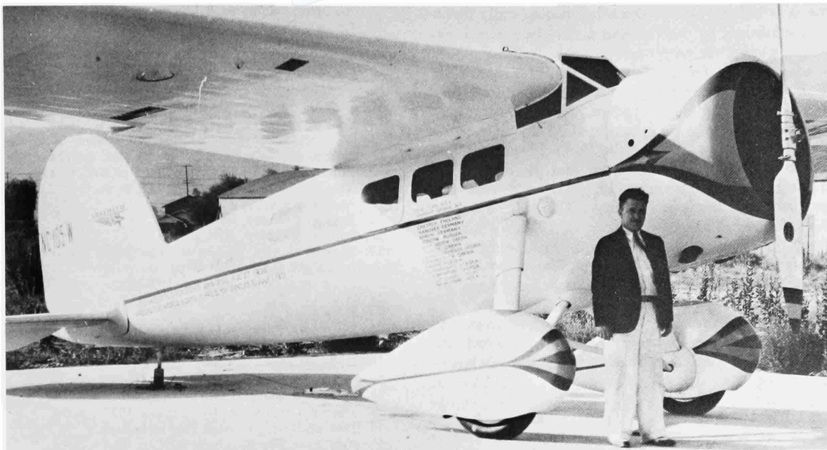
FIGURE 41. —Wiley Post stands before the beautifully reconditioned Winnie Mae , August 1932, Burbank, California. The propeller is of the fixed-pitch variety, and the lower right wing sports a retractable landing light (the light and the other, in the left wing, was extended manually or by an electric motor). The airplane is now in the “commercial” category (NC 105W). Note that the listing of the 1931 landings is lined up on the left margin, and that the exhaust is emitted at the lower side of the cowlings. The Winnie Mae is on a “compass rose” at the airport. (Courtesy Lockheed Aircraft Company.)
