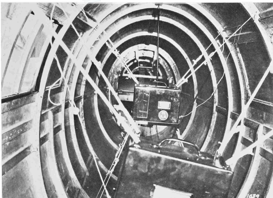
FIGURE 88.—This is a photograph showing the fuselage interior of Winnie Mae , with the two National Aeronautic Association barographs in place. Post's official altitude-record attempts were made, using this internal arrangement. The barographs were required to match one another within a prescribed tolerance. On the far barograph the recording pointers can be seen. Also seen are the security wire and its two sealing fasteners on the right side of the picture, attaching the rearmost barograph to a longitudinal metal support of the wooden fuselage. In the altitude attempt at Bartlesville, Oklahoma, on December 7, 1934, Post reached an unofficial altitude of approximately 50,000 feet. This could not be confirmed by the Bureau of Standards because one of the two required barographs failed to function. On this flight, Post discovered 200-mile-per-hour winds and confirmed his theories about the existence of high winds in the stratosphere. Post was the first pilot to fly in the "jet stream." (Courtesy Phillips Petroleum.)
