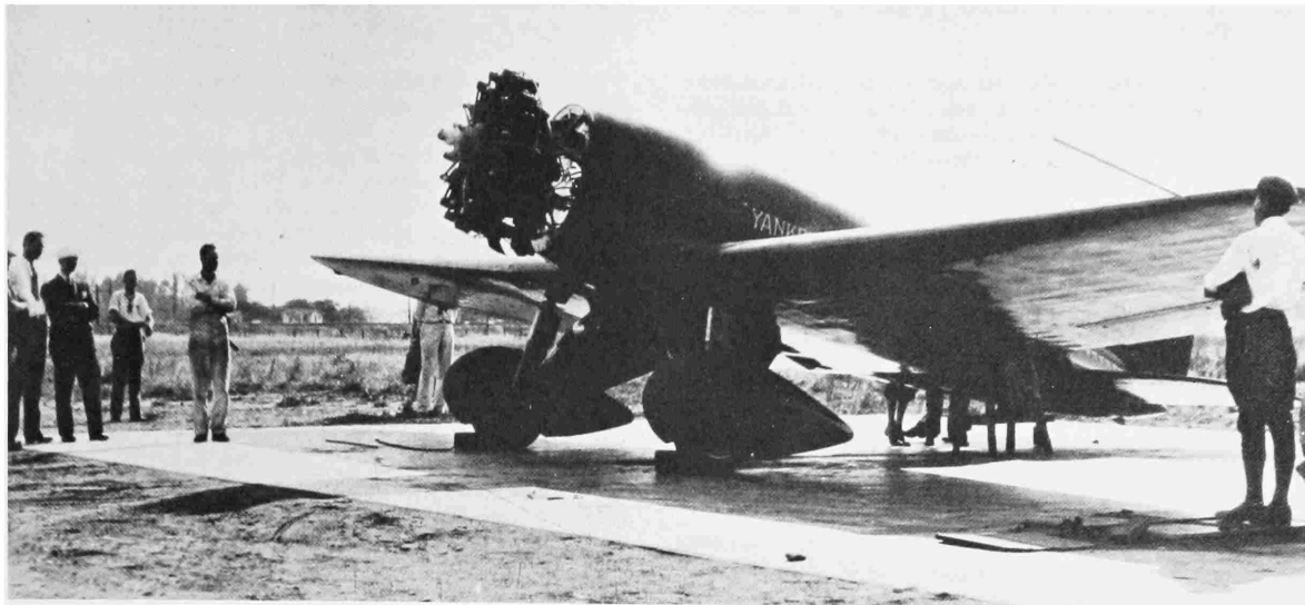
FIGURE 120.—The “Yankee Doodle,” a specially constructed Lockheed Explorer, is tested on June 3, 1930, at Los Angeles, California, during preparations for a planned Paris-to-New York, nonstop flight. Arthur Goebel hoped to fly the aircraft in the east-to-west direction, to be the first to do so. This airplane, license number NR 101 W, had a gasoline capacity of 800 gallons. Goebel did not take the plane but the Pure Oil Company did, and it set a nonstop record from New York to the Canal Zone. On November 21, 1930, the airplane was damaged in an accident at the Canal Zone and the wing was salvaged by Charles Babb. This wing was used with an Orion fuselage and became the hybrid aircraft that Post and Rogers flew to Alaska. (Courtesy Pacific and Atlantic Photos.)
