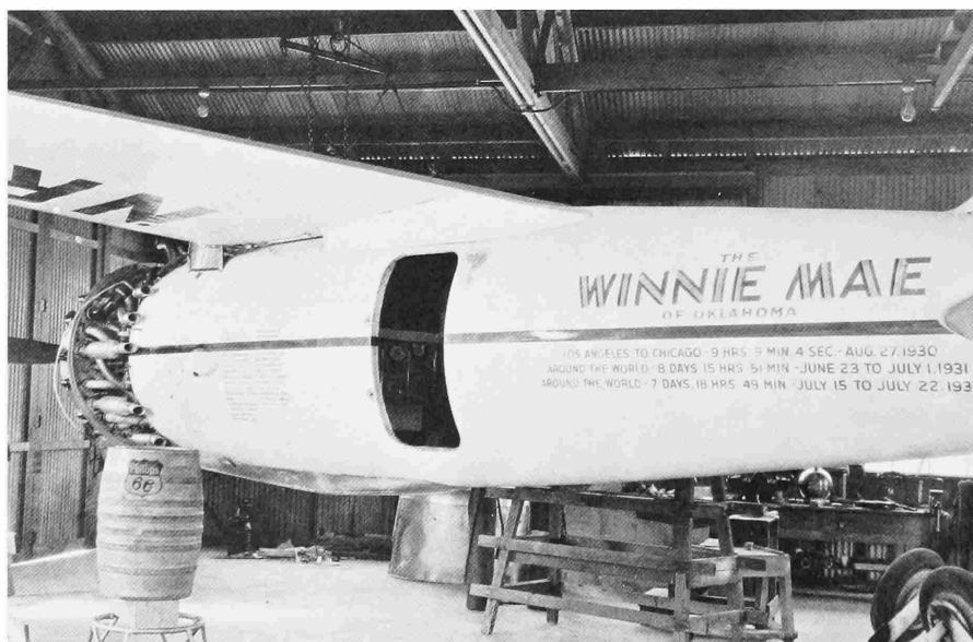
FIGURE 96.—The Winnie Mae is shown being prepared for a transcontinental stratosphere flight. This photograph was made in January 1935 at the original Lockheed hangar in Burbank. This hangar had been a "glass factory" prior to its use by Lockheed. The cowl has been removed and cleaned of paint (seen on floor behind fuselage). The aircraft is suspended by pullies from a ceiling beam by utilizing the hoist eye hooks on the upper wing. The belly-landing skid made of spruce has been glued in place and is now metal clad. Under the rear fuselage in the background on the workbench is the spherical container for the liquid oxygen. (Courtesy Phillips Petroleum.)
