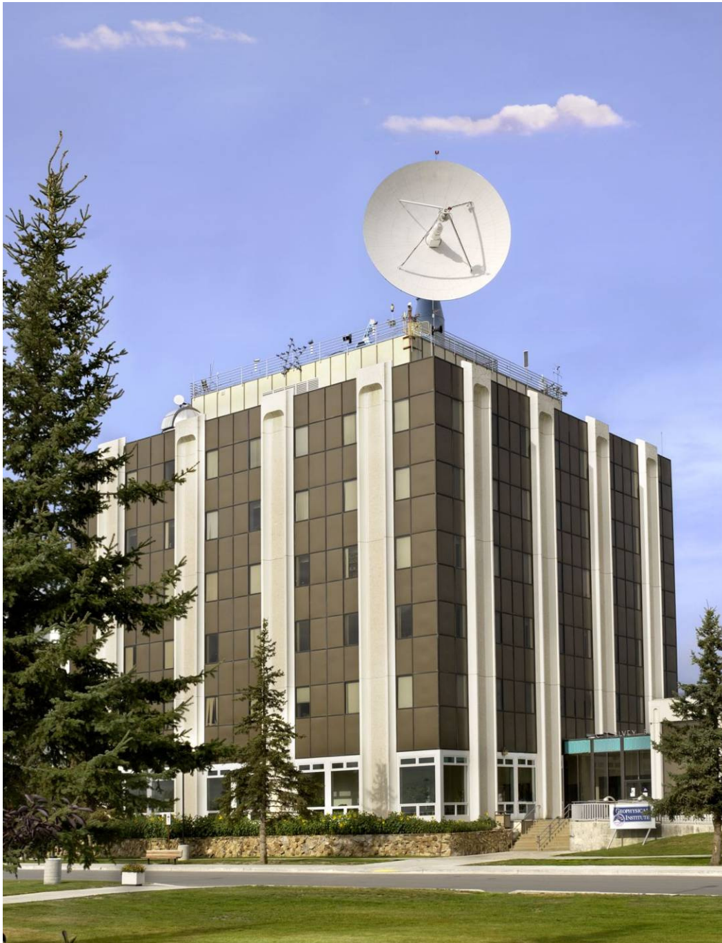
Figure 7-1. ASF 10-meter Antenna
