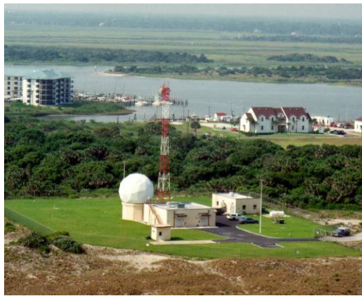
Figure 8-2. PDL Ground Station
