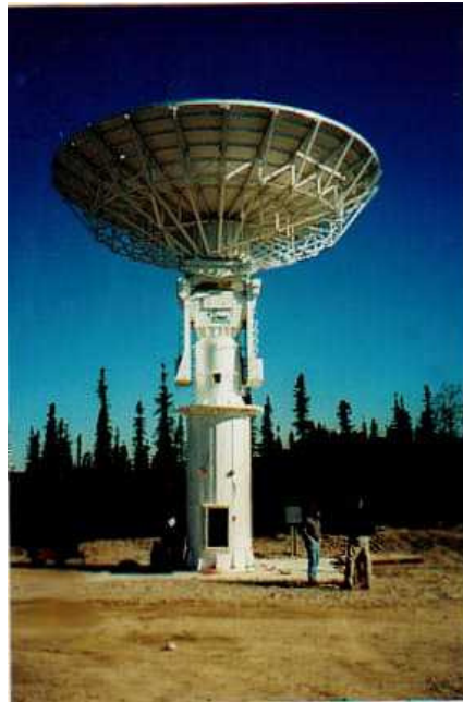
Figure 6-2a. PF2 Antenna Before Radome Installation
