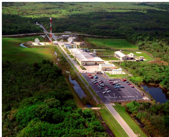
Figure 8-1. MILA Ground Station
