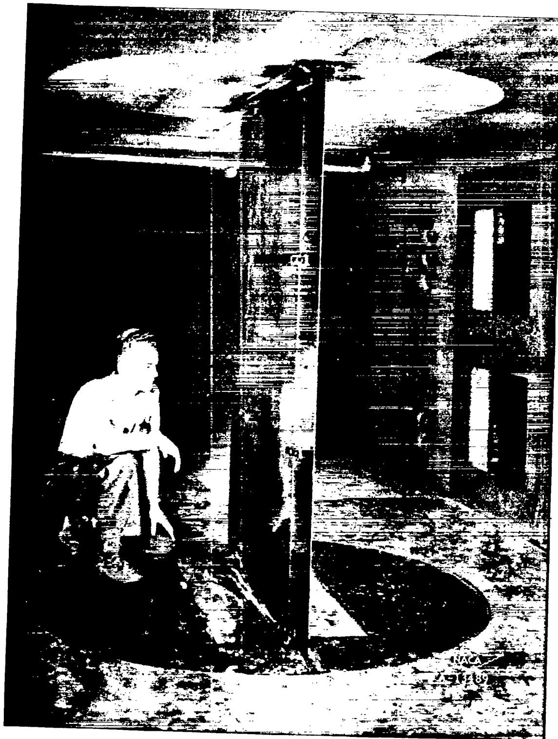
Figure 2.- The faired, double-wedge airfoil model installed in the wind tunnel.
