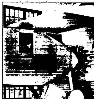
FIGURE 12.—Cowling No. 4, engine exposed
