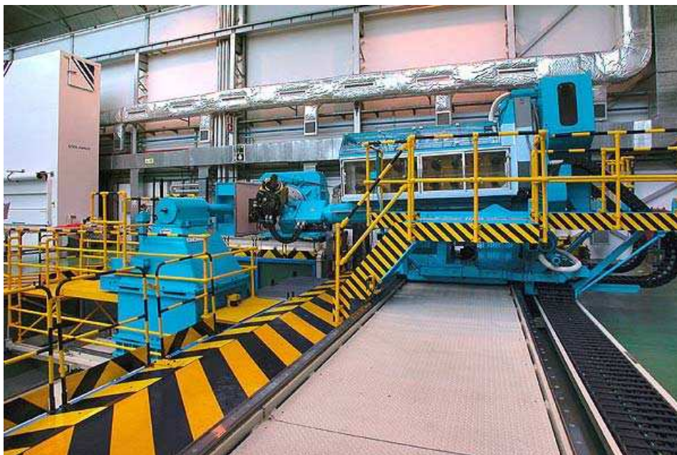
Figure 38.14-3 – Fibre placement: General view of working area
