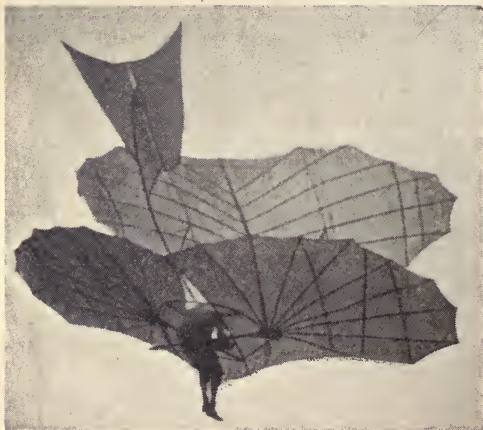
FIG. 2.—Lillienthal's biplane glider in flight, 1894.
