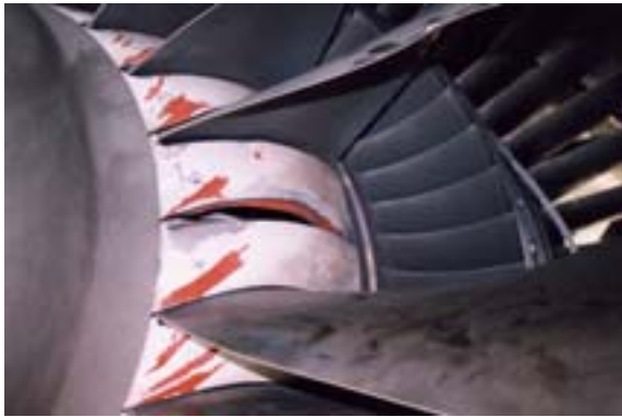
Fig. 3. View showing the fan rotor annulus filler plates around the failed blade position.
