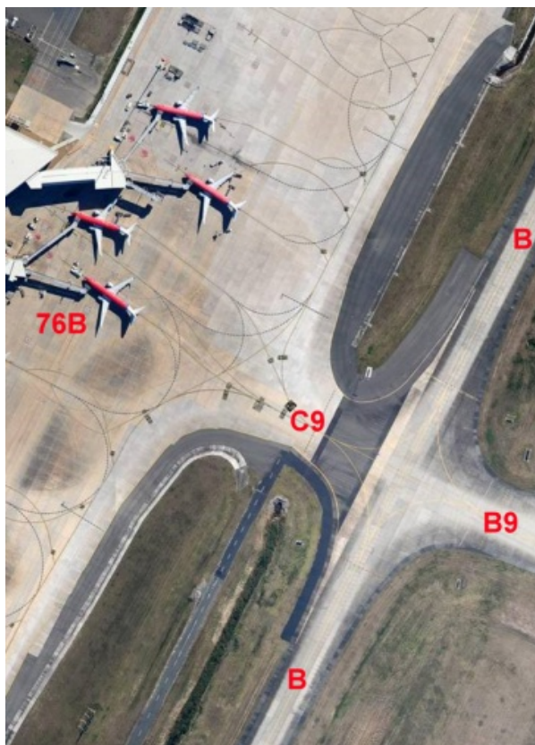
Figure 1: Parking Bay 76B and Taxiway C9
