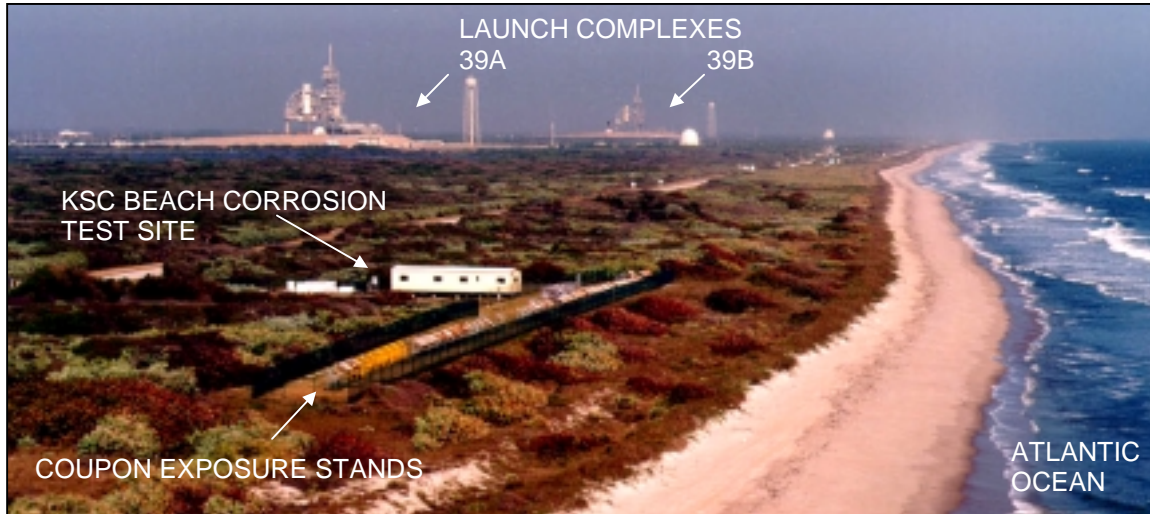
FIGURE 3: View of Beach Corrosion Site and Coupon Stands
