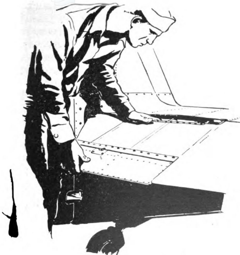
Figure 58.—Adjusting elevator tab.
