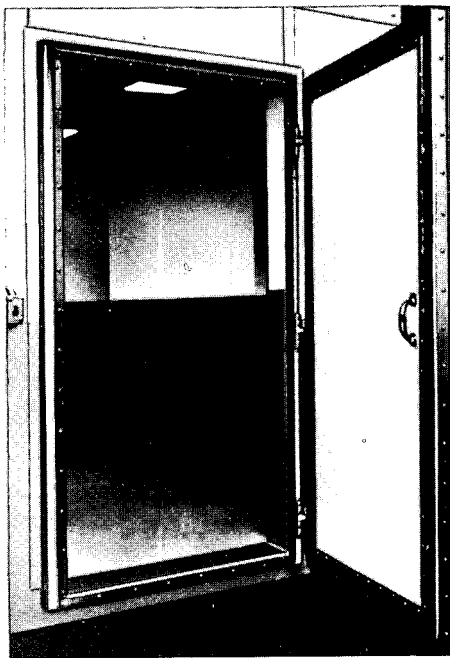
Fig. 4-76 Entrance to r.f. shielded room
