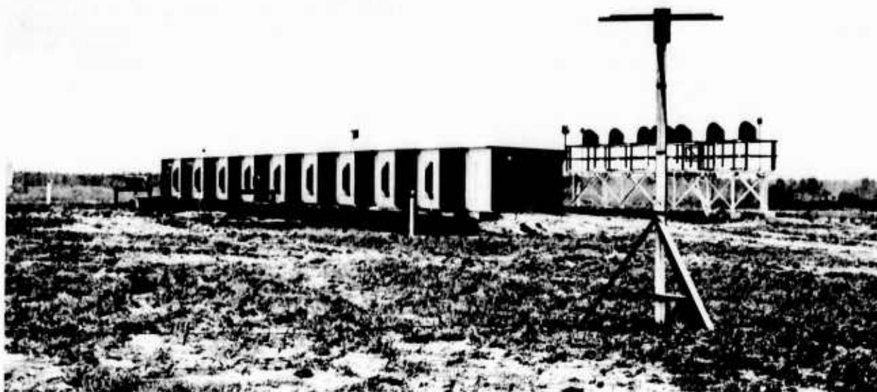
Figure 4.4 Wave-Guide Localizer Showing Clearance Array and Monitor Probe
