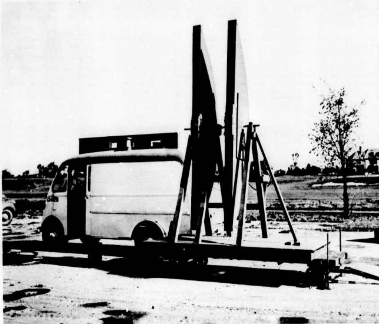
Figure 2.1 Early 3000-MHz Sperry Microwave Glide-Slope System (about 1942)
