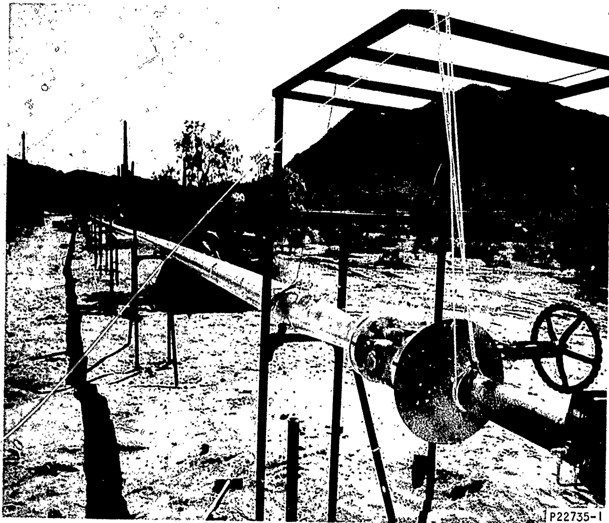
Figure 78. Pump Discharge Control Valve and Dump Line
