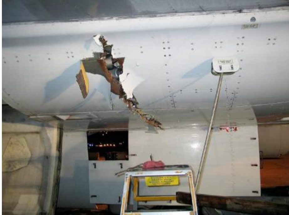
Figure F16: Photo of B747 Fuselage with Disk Penetration Damage Caused by Uncontained Rotor Failure
