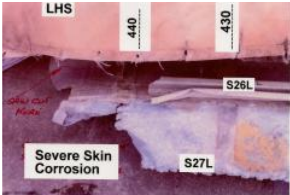
Figure D5: Photo of Skin Corrosion in Lower Lobe of B737 Aircraft
