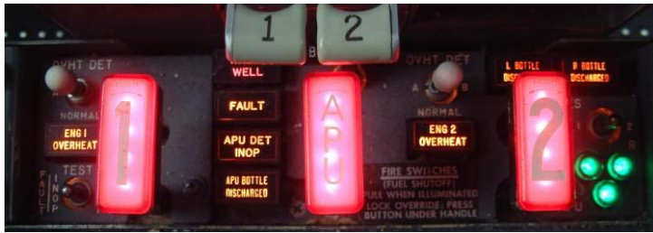
(Photo of cockpit fire panel above is from the “737 web site” and used with permission by its author, C. Brady.)
