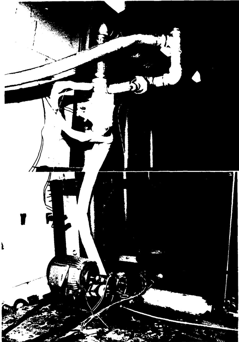
Figure 4-18, A Bypass was Used on the Heater for the "Coolant" Flow
