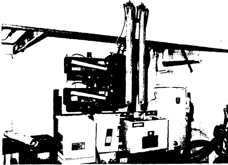
Figure 4-15, The Manometers for the ASME Flow Nozzles
