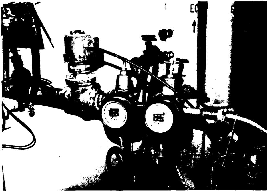
Figure 4-17, Dual In-line Pressure Regulators
