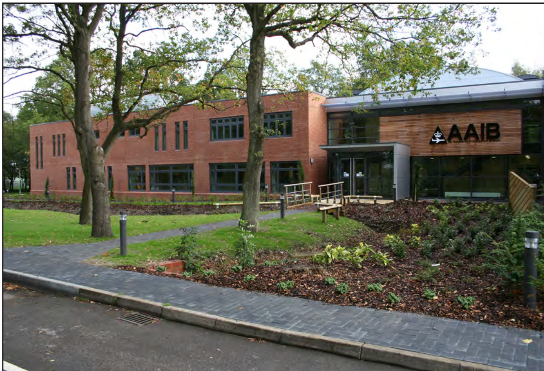
AAIB HQ at Farnborough
