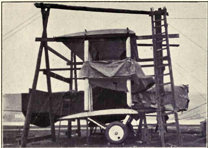
FEATHERING THE WINGS—SETTING UP THE FLIER AT ST. JOHNS, N. F.
