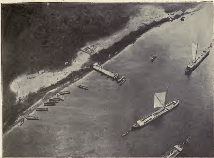
FIG. 144.—Building a pontoon over the Spree.
