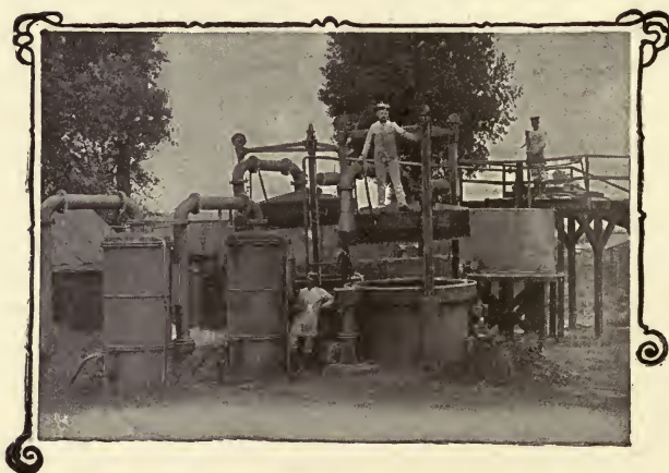
FIG. 92.—Old method of generating hydrogen.
