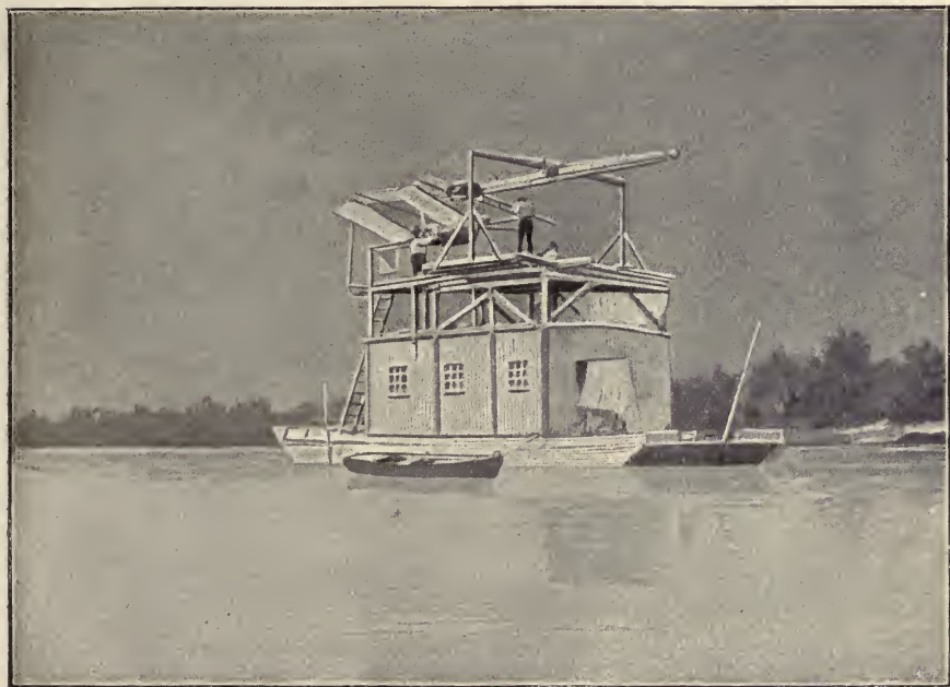
FIG. 56.—Starting arrangements for Professor Langley's flying machine.
