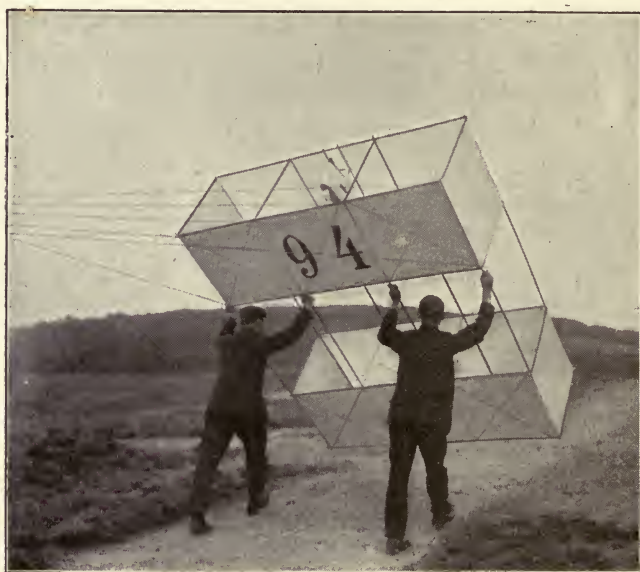
FIG. 161.—Ascent of a box-kite containing meteorological instruments (Photograph by the Berliner Illustrationsgesellschaft.)
