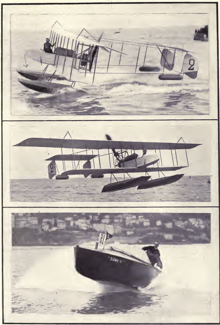
The Henry Farman hydro-biplane, about to rise and about to alight. Below is a fast flat-bottomed motor-boat, showing how the bows rise from the water at high speed.
