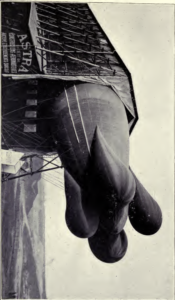
THE "BAYARD-CLEMENT" ENTERING ITS SHED, SHOWING THE PNEUMATIC ENPENAGE
