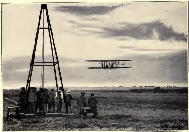
THE WRIGHT AEROPLANE AT THE MOMENT OF LAUNCHING BY THE DROP OF A WEIGHT FALLING FROM ITS "PYLON"
