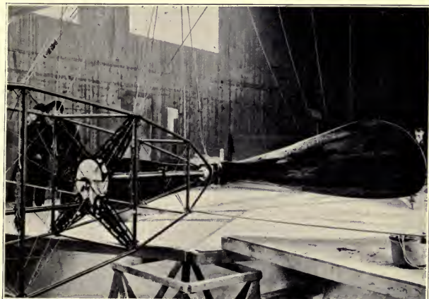
THE SCREW-PROPELLER OF THE "BAYARD-CLÉMENT"
