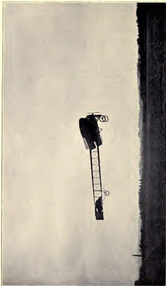
LOUIS BLÉRIOT'S MONOPLANE IN FULL FLIGHT (THE FOSTER-CLASSIS AND THE "AILERON" AT THE TIP OF EACH WING ARE PLAINLY SHOWN) Photo, Branger
